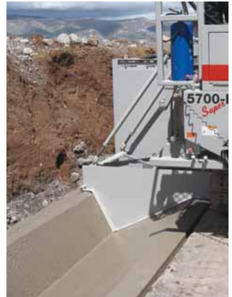
V-Ditch, 5' (1.5m) wide and 20" (.5m) deep in Peru.
