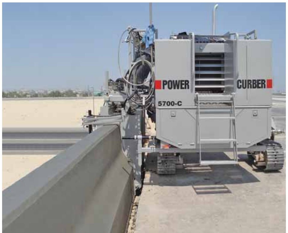
Barrier poured below grade, 49" (1.25m) tall.
