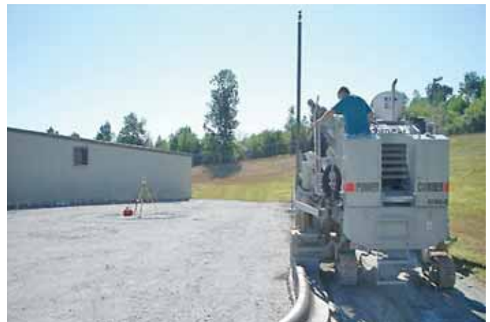
Pouring curb & gutter with 3-D (stringless) control.
