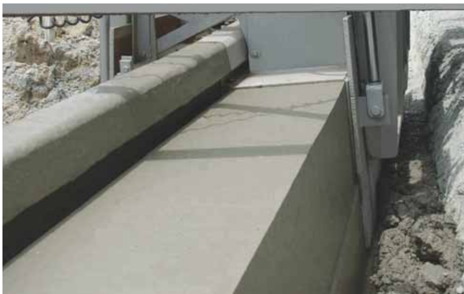
Slotted drain poured below grade.
