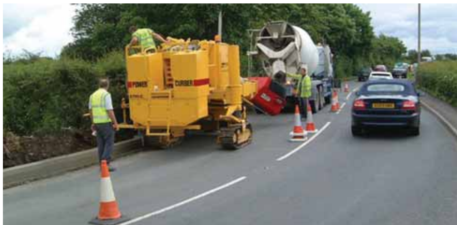
Single lane pouring minimizes traffic interruption.
