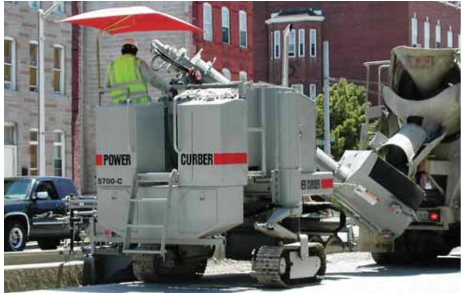
Barrier Curb in a rehab application, working on a crowded city street.
