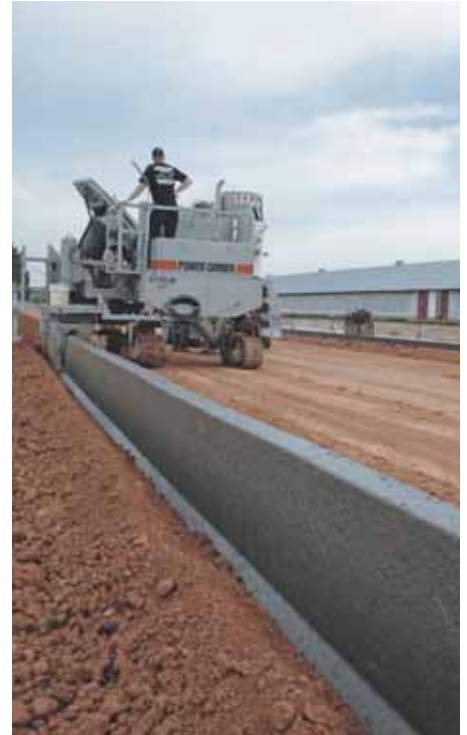
Poultry house foundation poured over trench.
