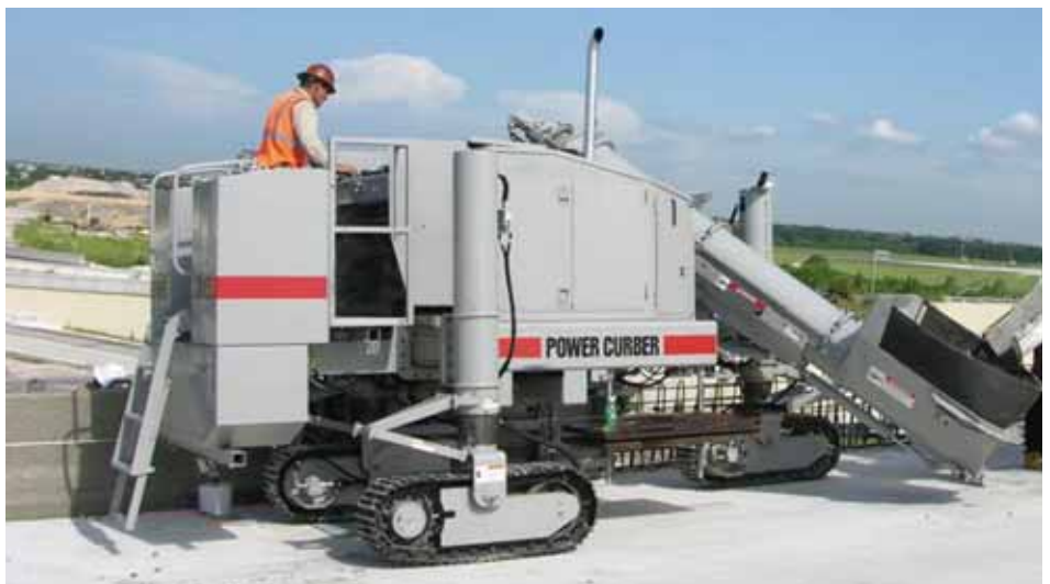
5700-C pouring bridge parapet in Florida.
