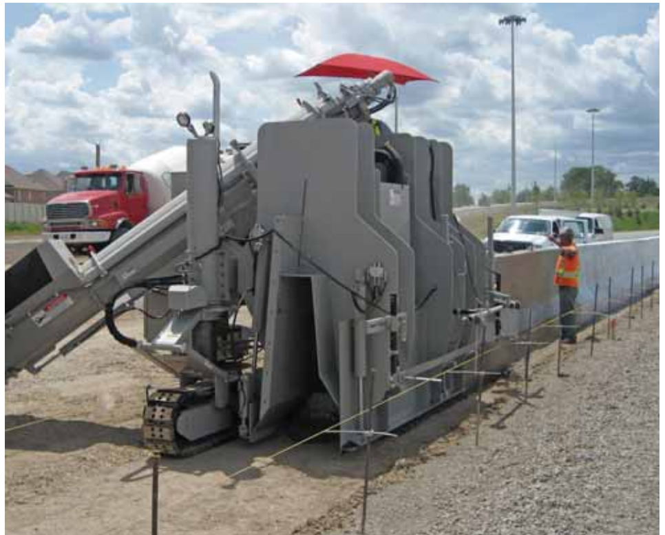
5700-C-MAX pouring large variable barrier wall.
