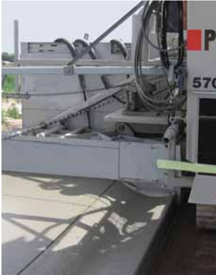
Monolithic curb, gutter, and sidewalk.
