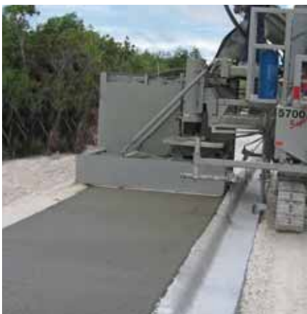
Sidewalk adjacent to back-of-curb. Sensing off-curb.
