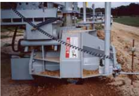
Custom trencher trimmer for footings.
