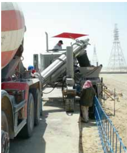
Barrier below grade with rebar.
