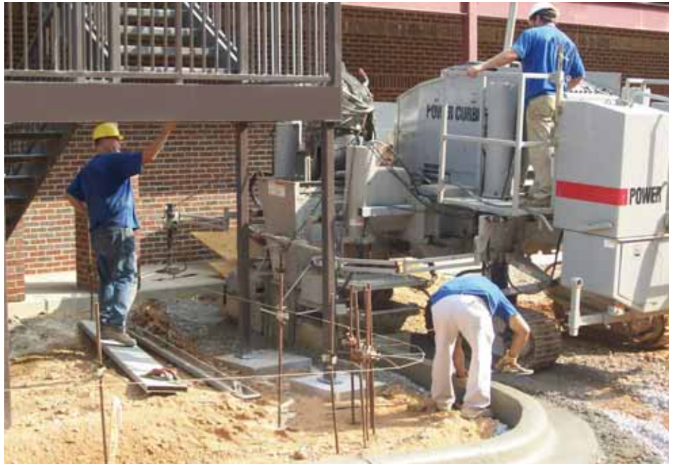
Machine maneuvers in tight areas, minimizing tie-ins.
