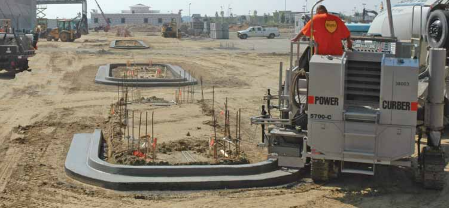
The machine's tight radius capability eliminates hand forming parking lot islands.
