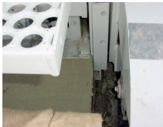
The side-forms are connected to the tracks.
