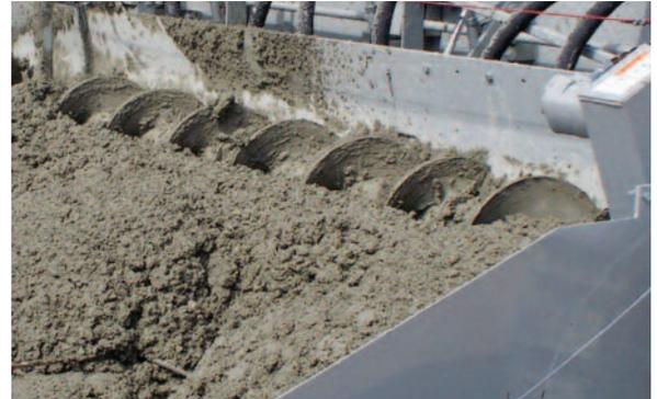
The spread auger and strike-off plate.
