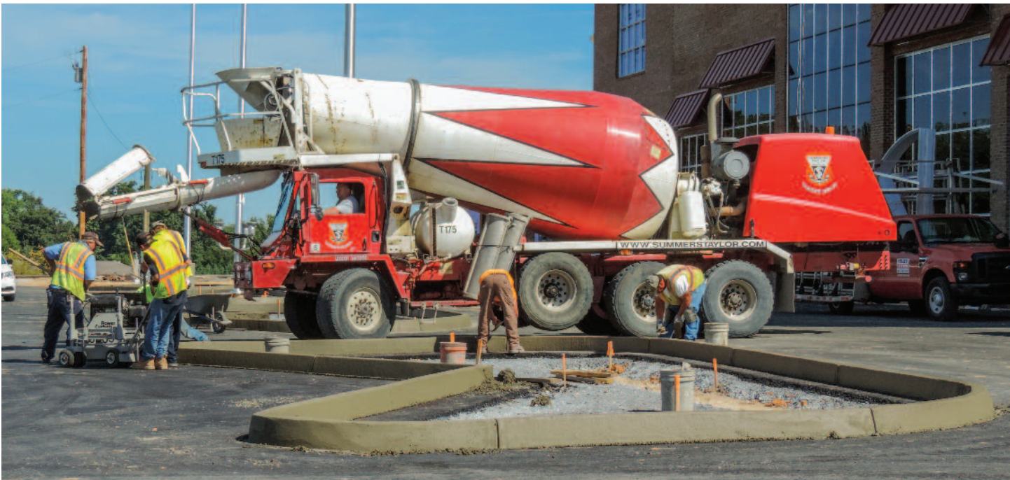
For jobs that require less expensive scab-on curb, extruded curb can be the ideal solution.
