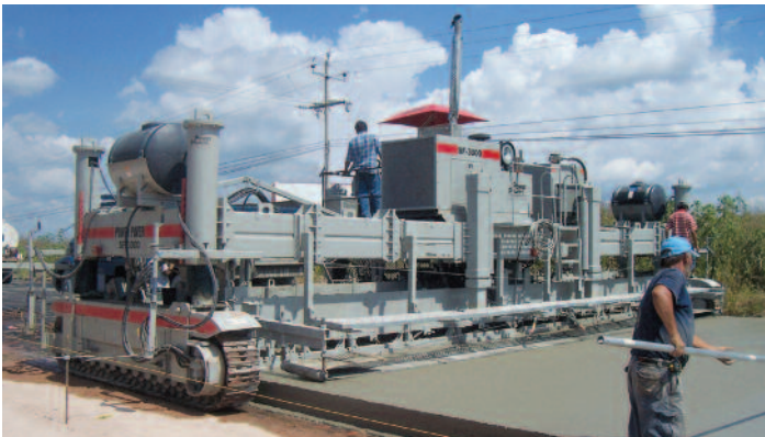
▲ Power Pavers SF-2700 and SF-3000 Slipform Pavers
