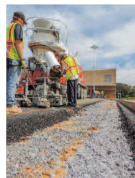
The 150 can pour clean, straight curb on a subgrade of 95% compaction, or on existing pavement.
