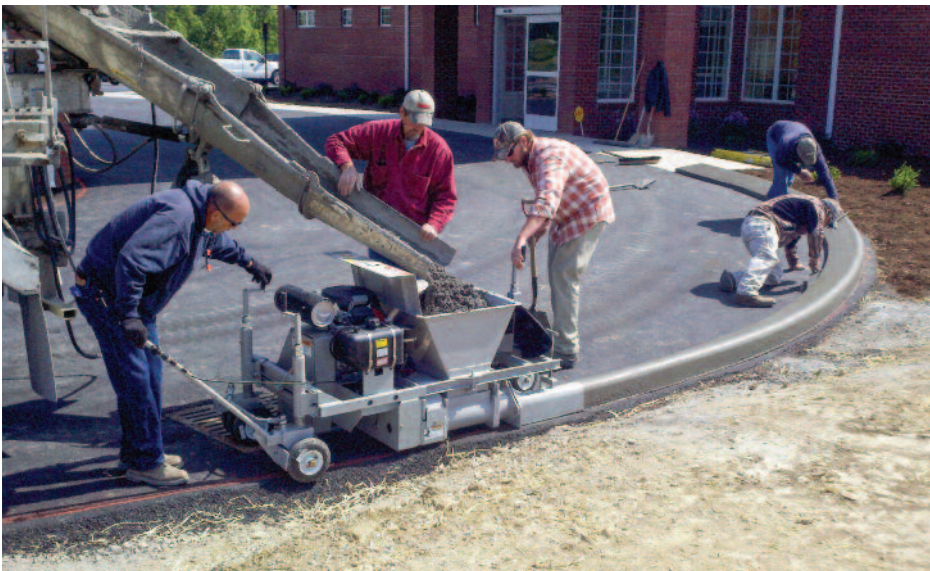
The extrusion process propels the machine forward.
