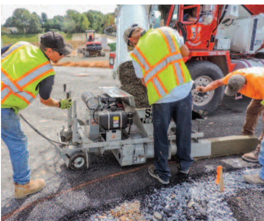
Three lifting jacks make adjusting on the fly quick and easy.
