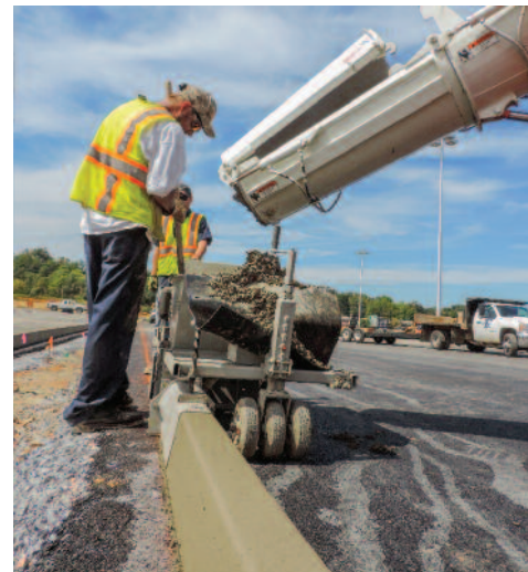
The 150 is easy to operate; one person steers while another ensures that the concrete or asphalt is reaching the auger.
